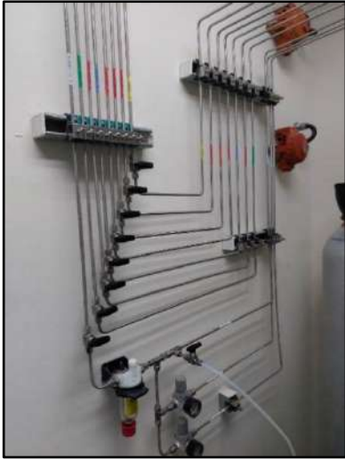
Figure 3.2 Main Supply Gaseous
